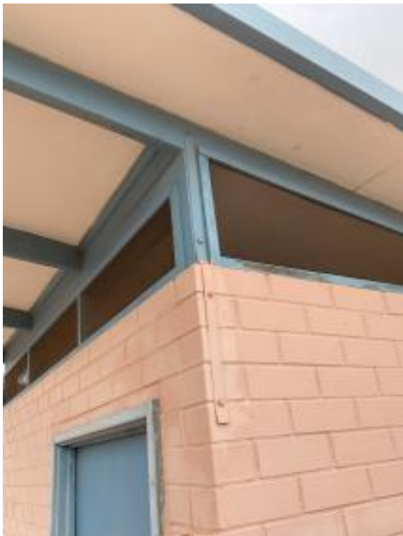
Insufficient tie-down
