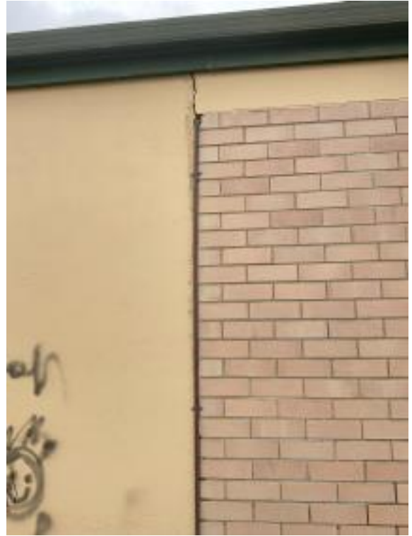
Separation between Filter Tank and Plant Room
