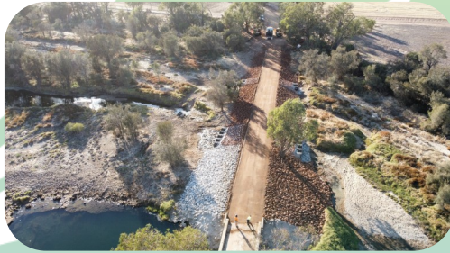
Mackie Siding Bridge Repairs
