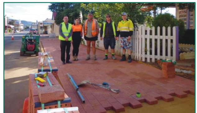
Avon Terrace Footpath
