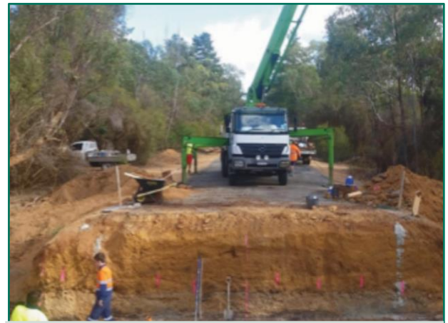
Talbot Road West Bridge Replacement
