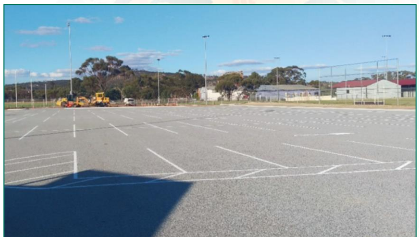
York Recreation and Convention Centre Carpark
