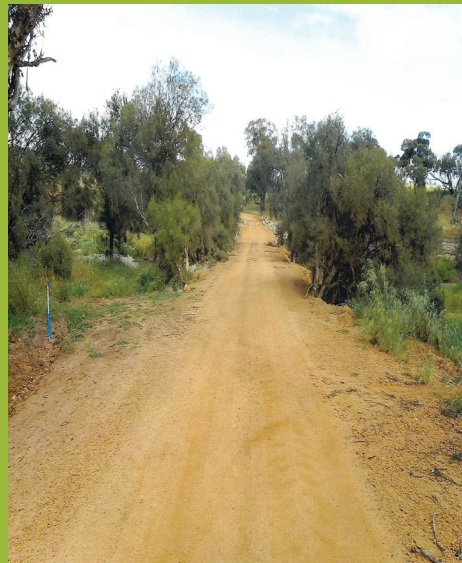
After repairs – Mackie Siding Road
