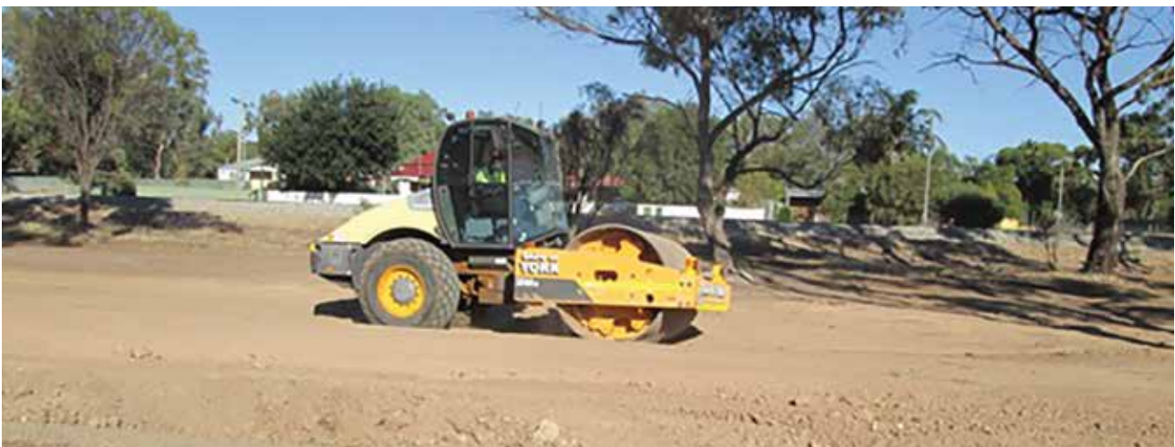
Avon Terrace drainage completed
