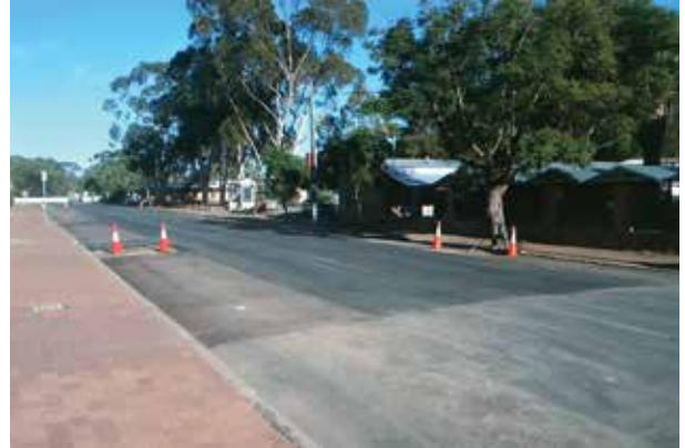
Joaquina Street seal completed
