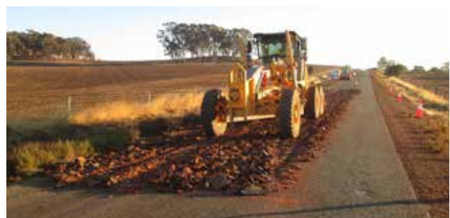
Qualen West Road Pavement Repair
