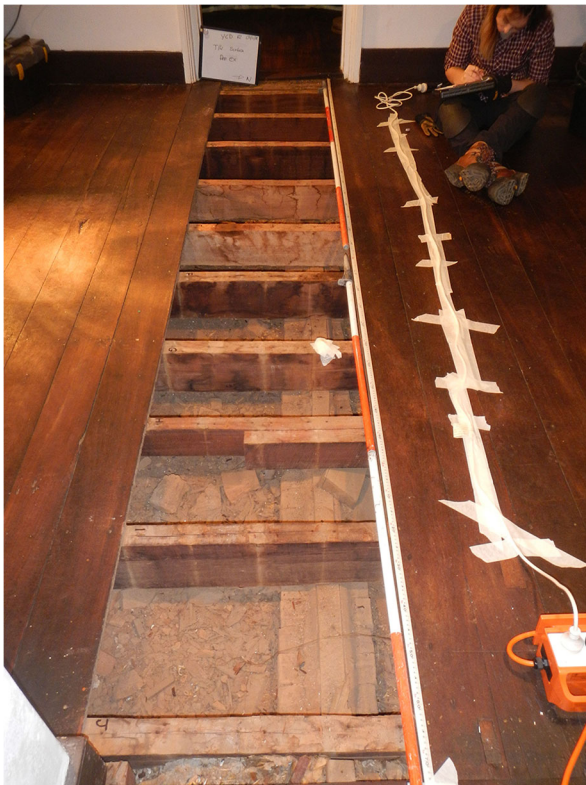
Fig. 5 Excavation trench at the York Residency Museum (photo S. Winter)
