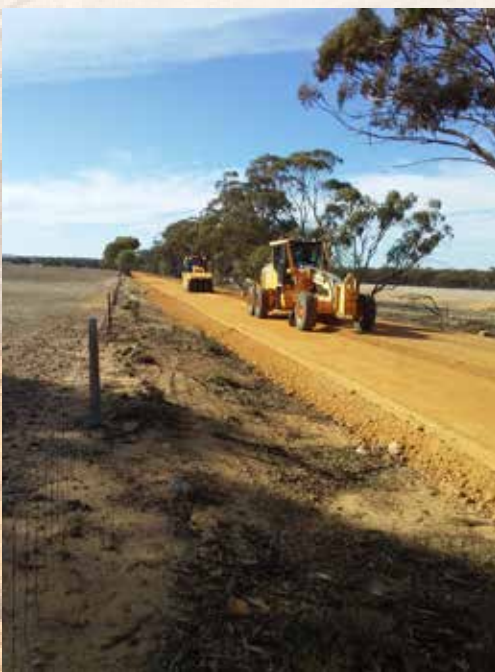
Depot Goldfields roads re-construct
