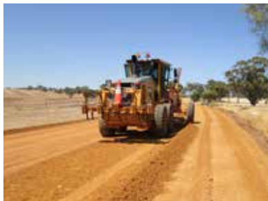
Mannavale Road reconstruct & widen
