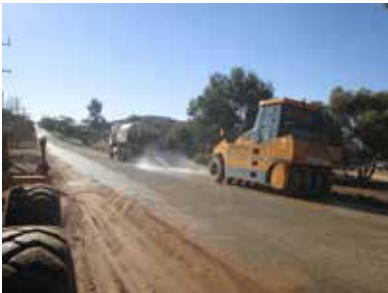
Tenth Road widen seal kerb
