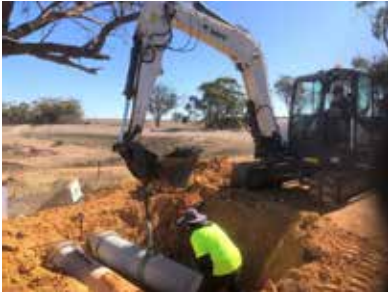
Greenhills South Road drainage
