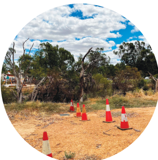
Drainage improvements made at RV Park on Janet Millet Lane
