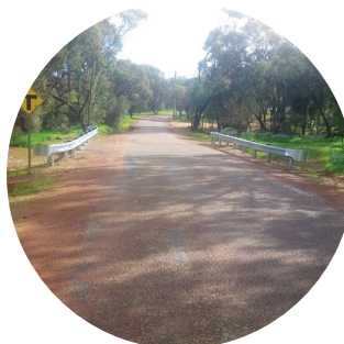
Construction clearing culverts and drains
